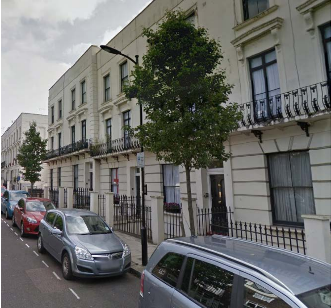
Front elevation of Nos.16-18 Blomfield Villas.
